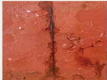
Prevent Corrosion Failure
